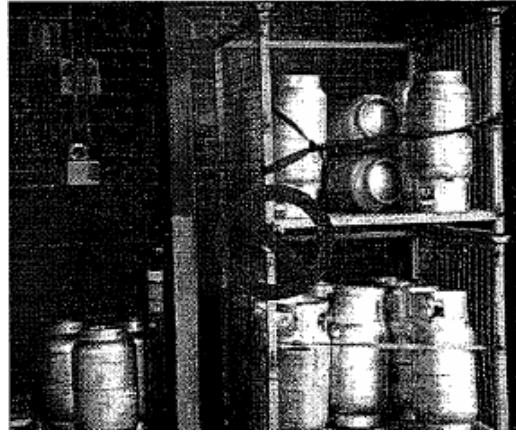
Cylinders should be stored in an upright position so the pressure relief valve is able to vent
